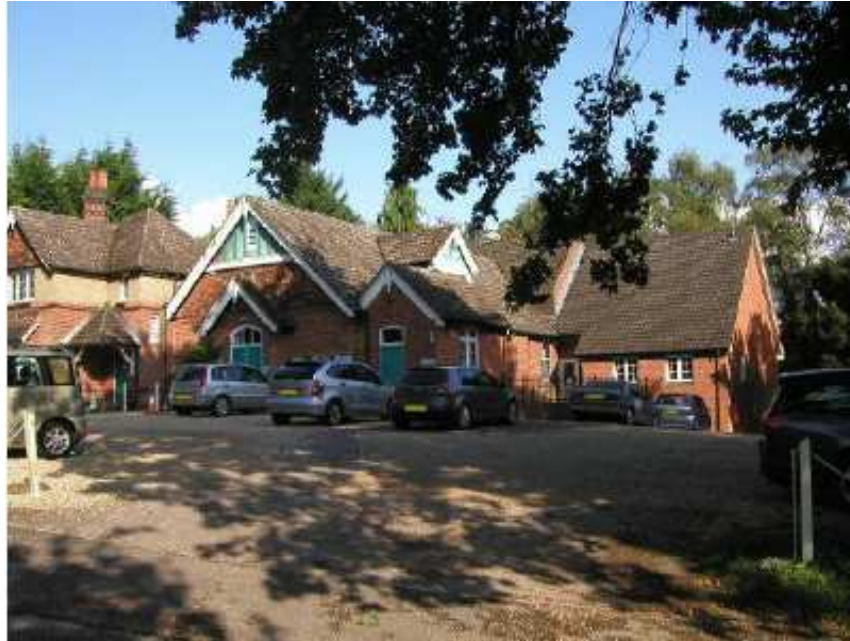
Shawford Parish Hall, Pearsons Lane, Shawford SO21 2AG
